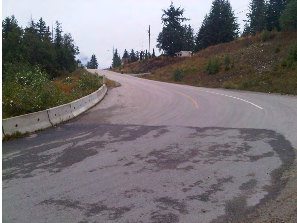
Figure 5-4 Vavenby Bridge - South Approach
