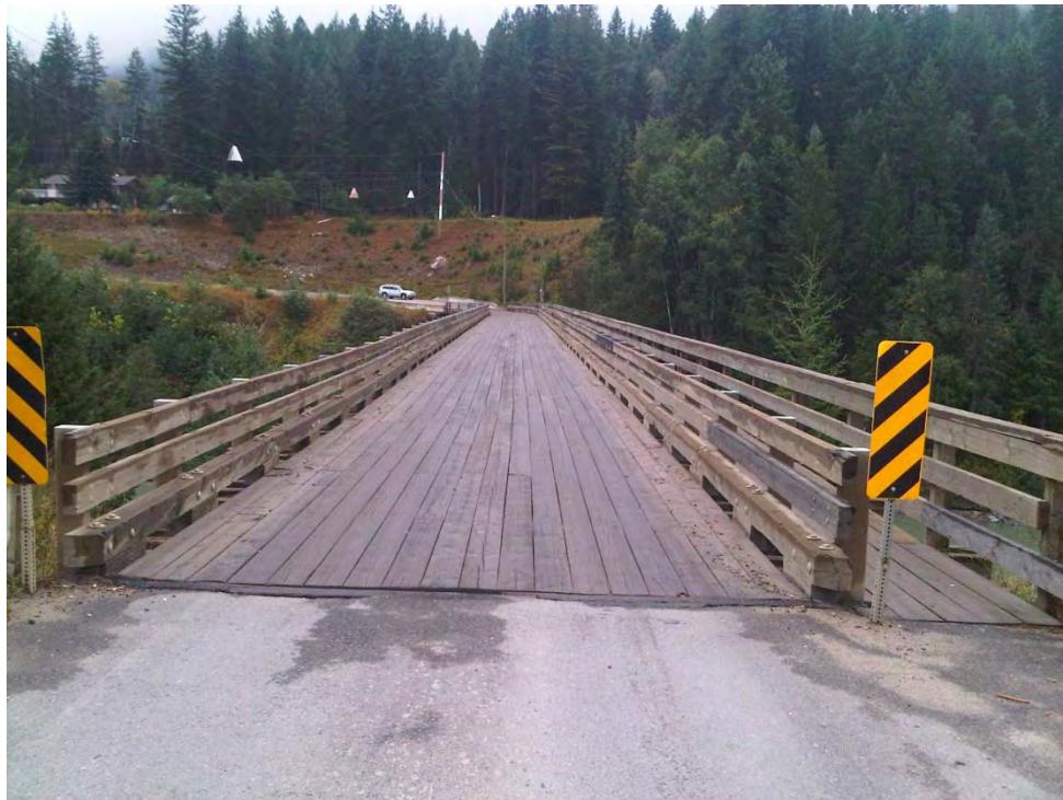
Figure 5-3 Vavenby Bridge - Looking South
