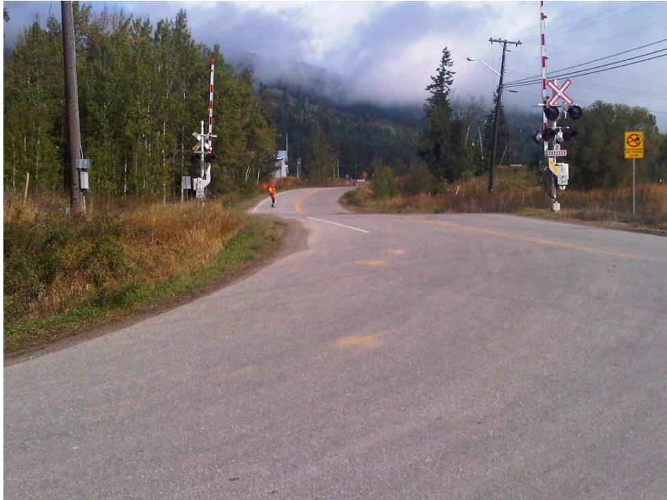
Figure 4-3 McCorvie and Vavenby Bridge Road - CN Crossing
