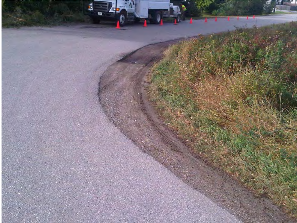
Figure 4-5 McCorvie and Vavenby Bridge Road - Truck over-tracking
