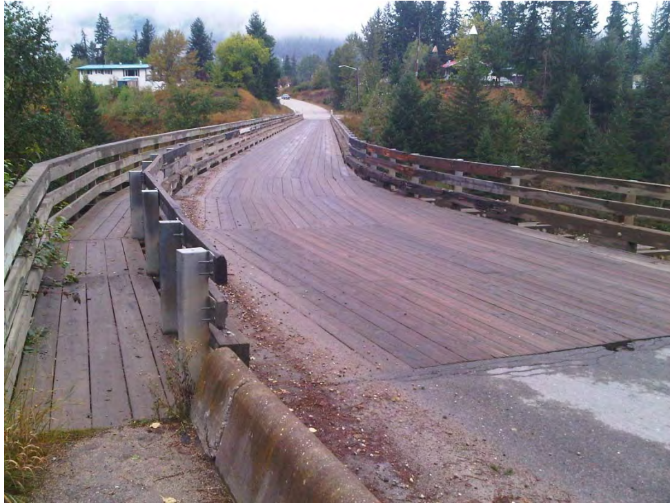
Figure 5-2 Vavenby Bridge - Looking North
