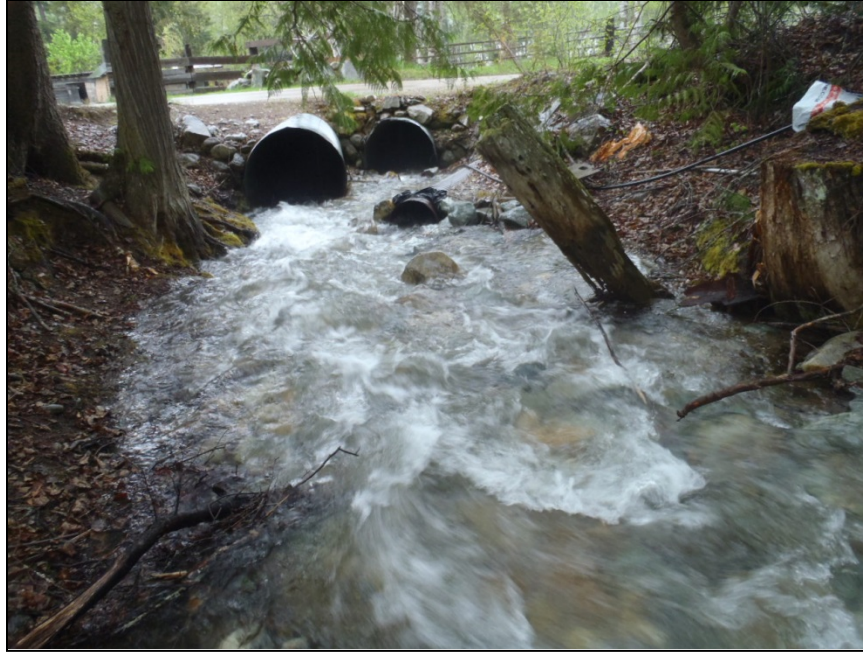
PHOTO A3 – Baker Creek hydrology station (BAKER), looking downstream
