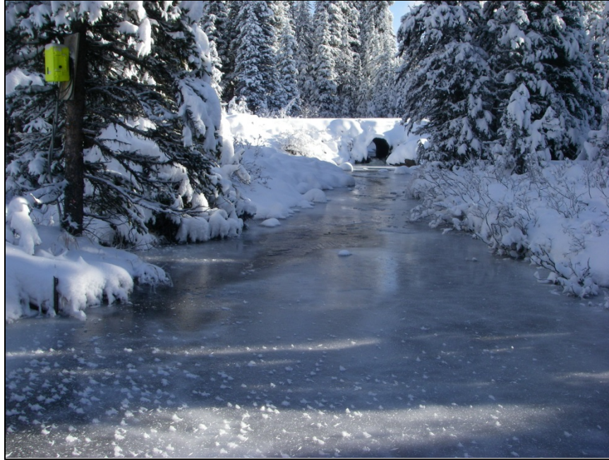
PHOTO I5 – T-Creek hydrology station (TSFUS), winter conditions
