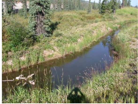
Photo 2. Looking downstream at typical habitat within the diversion channel.
