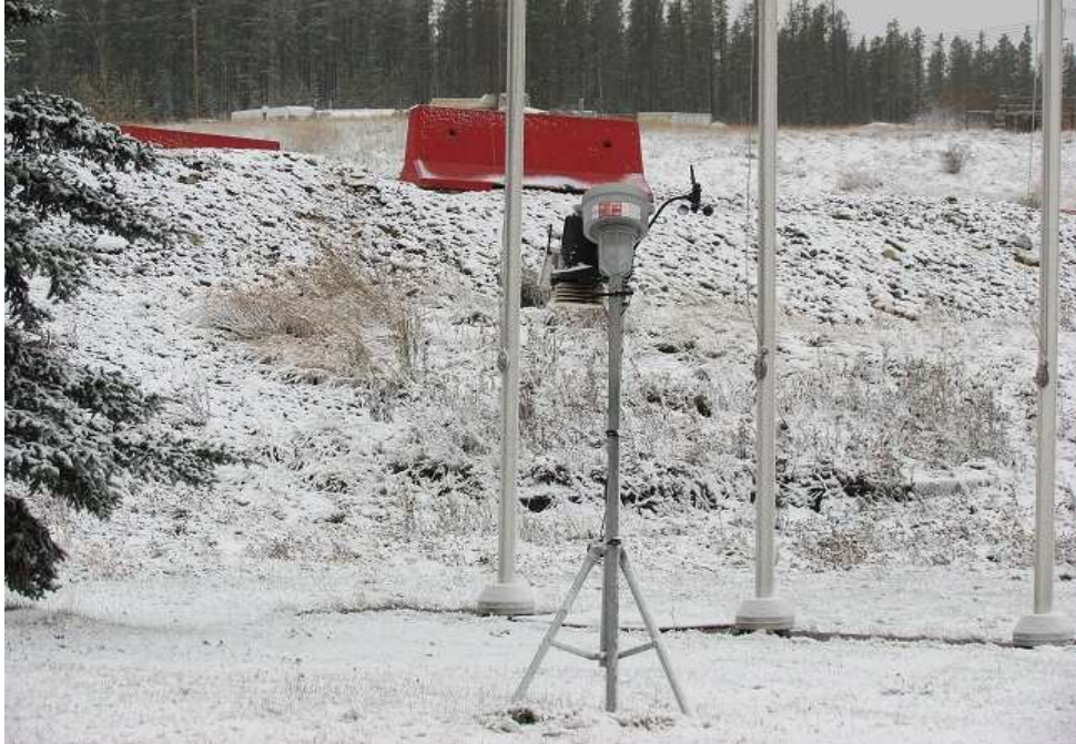
ESRD Photo 54-1 Wind Sensor Siting at the CVRI Coal Processing Plant
