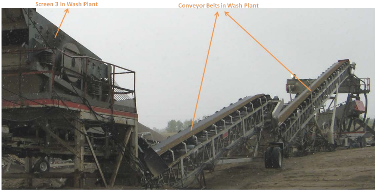
Photo 7: Wash Plant Conveyors
