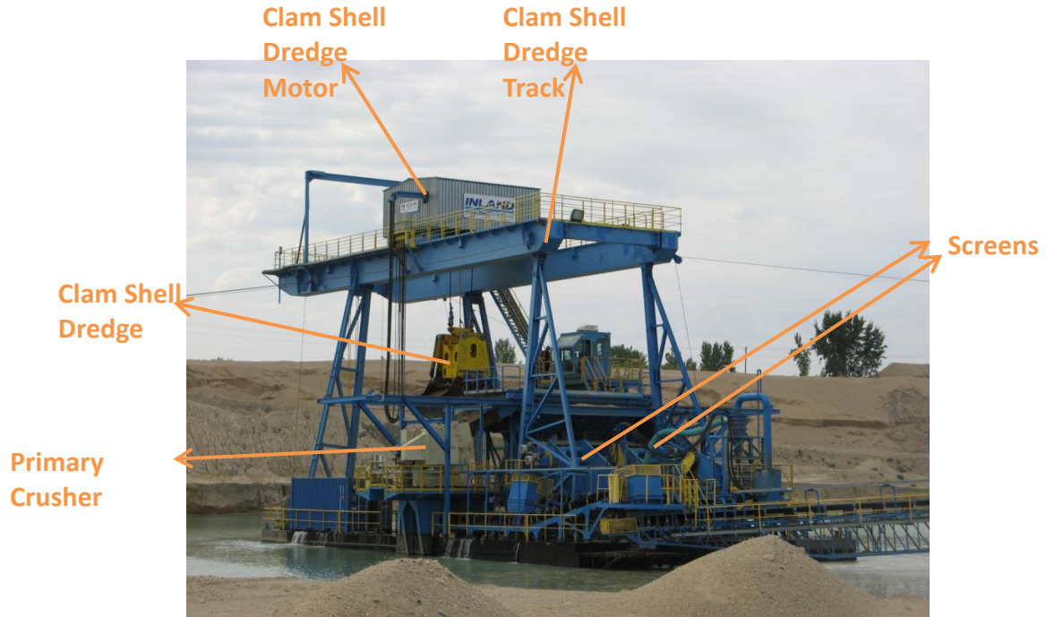
Photo 1: Floating Deck and Equipment on Deck
