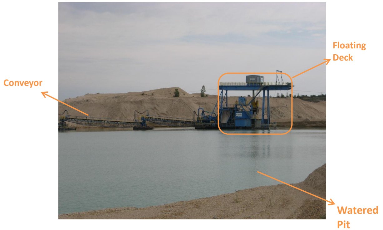
Photo 2: Pit, Floating Deck and Conveyor System
