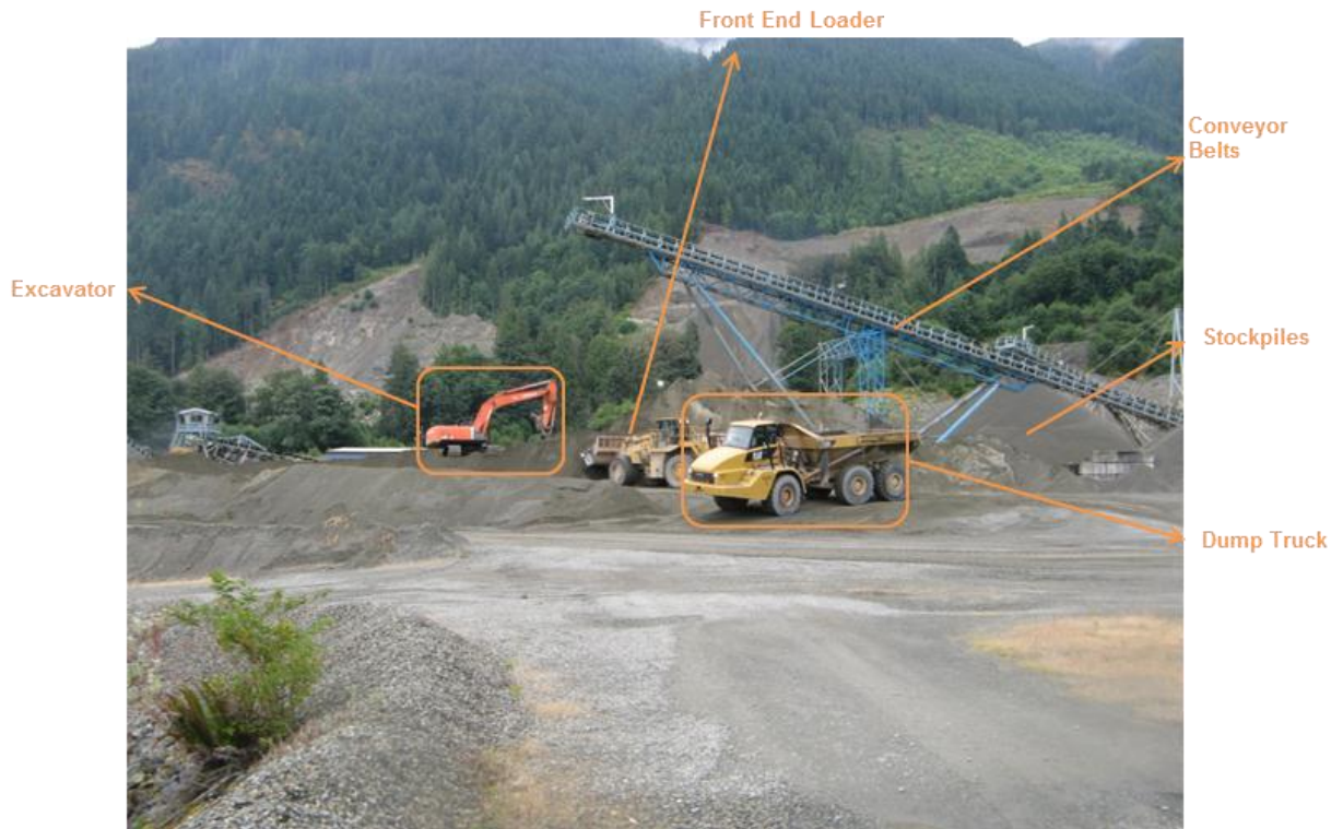
Photo 2: Sorting and storage area
