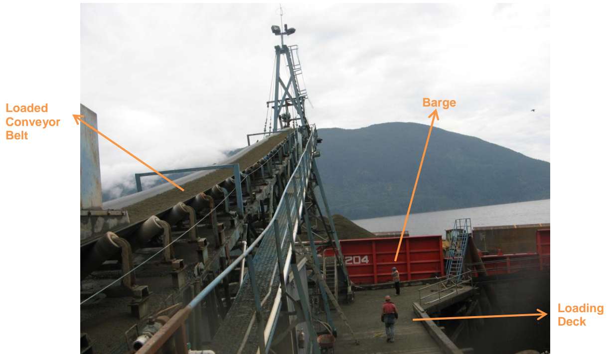
Photo 4: Barge loading area (looking out from the shoreline toward Jarvis Inlet)
