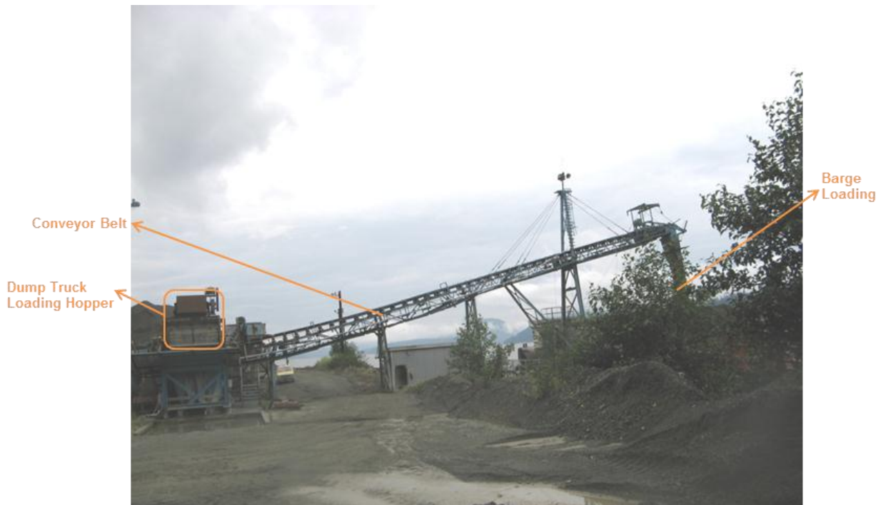
Photo 3: Barge loading area (looking parallel to the shoreline)
