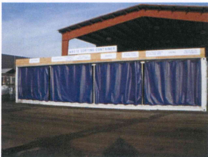
Temporary hazardous waste management area at Vancouver Shipyards Co. Ltd. (under construction in 2013/14)
