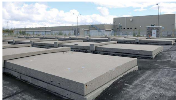
Figure 2-9: Trench Waste Storage Units
