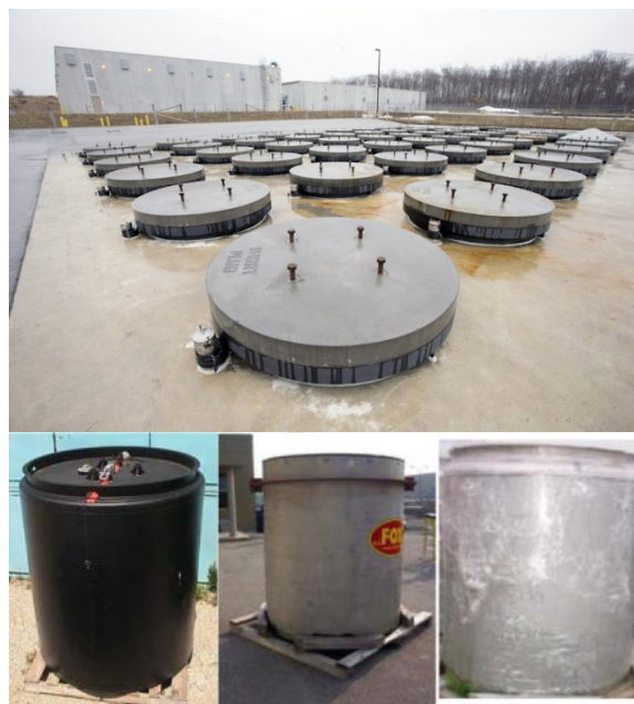
Figure 2-25: IC-18 Storage Units and Carbon Steel Resin Liner, Stainless Steel Overpack and Stainless Steel Resin Liner
