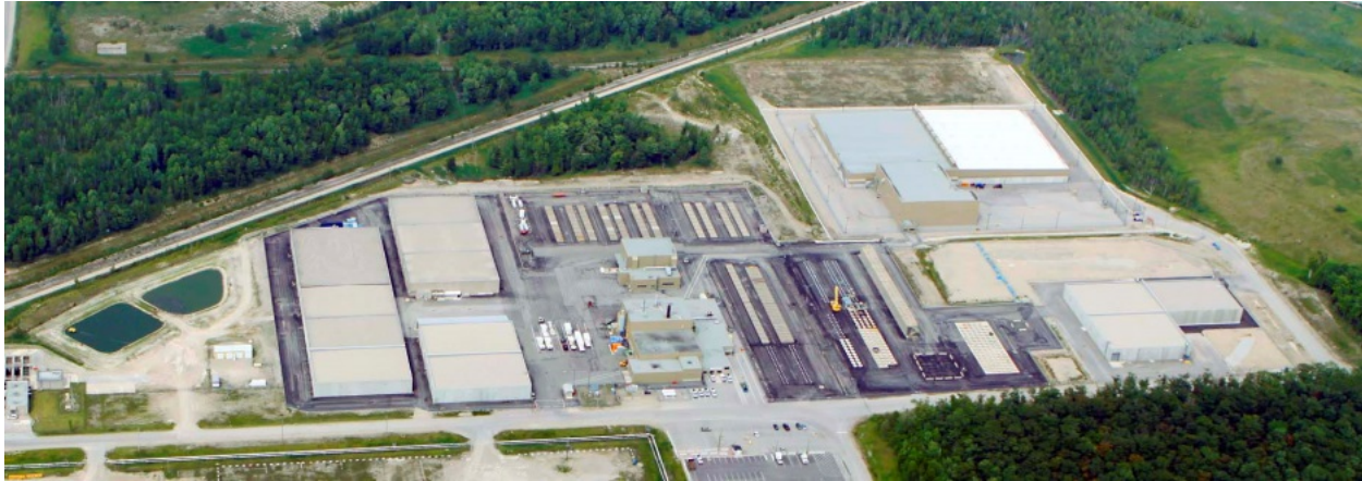
Figure 2-1: Aerial View of WWMF
