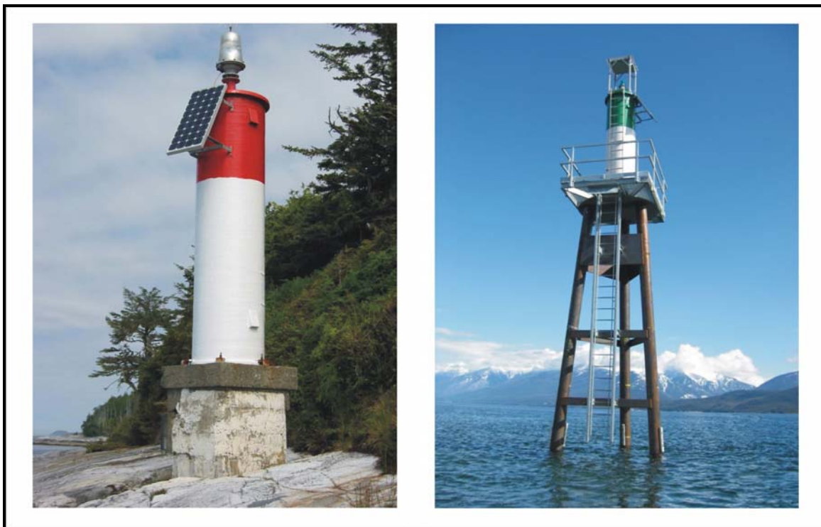
Figure 1: Typical concrete-based and pile-based RCSR structures
