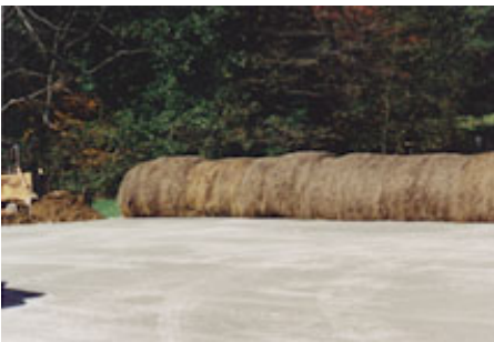
Figure 3.3 Photograph example of a storage pad constructed for hay bales
