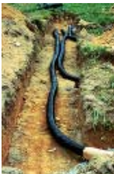
Figure 3.8 Photograph of trench and drainage lines
