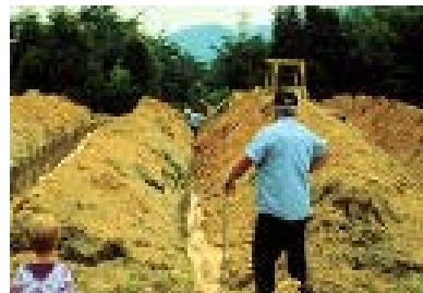
Figure 3.10 Photograph of the completion of treatment bed installation
